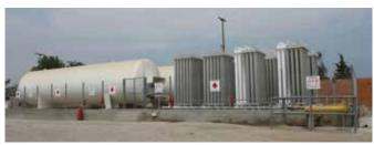
Complete LNG system 2 x 95 m³ LNG storage tank 8 pcs. ambient vaporizer
